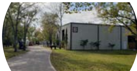
4 Drive past Building B Stay to the right of the fork
